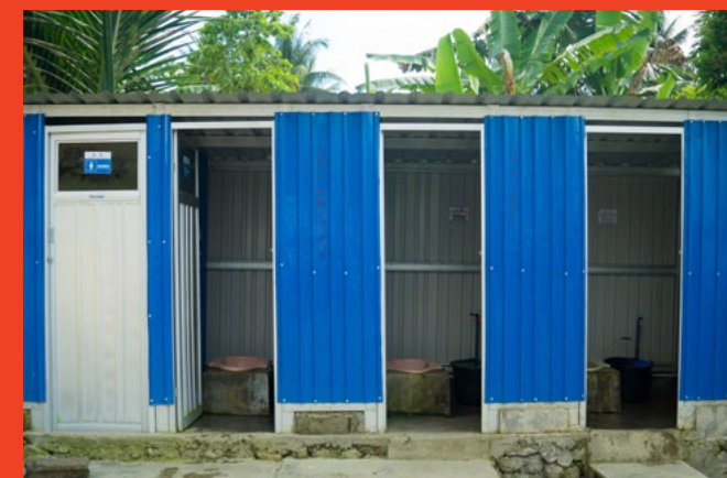
To make sure that more people had a sanitary and private toilet, we built 25 four-stall public toilets in 10 different villages and camps for more than 1,700 people to use. Then we turned our attention to helping families who were not permanently displaced build private toilets in their homes.
